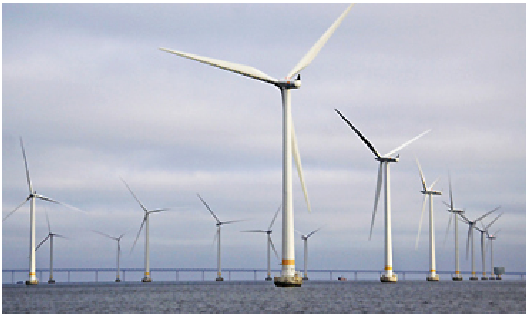
Figure 1: Wind Power at Lillgrund, Sweden.
